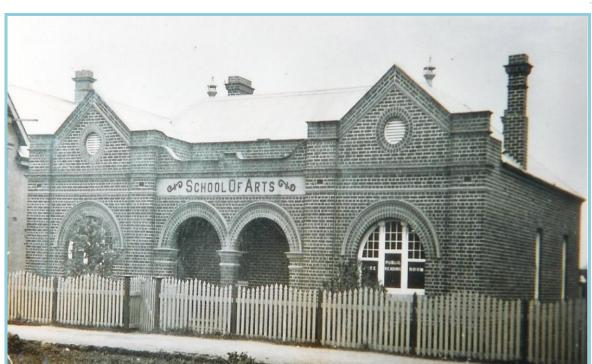
The present paint scheme disguises the strong red-brick character of the School of Arts. Many specially moulded bricks were used in construction. The handsome arched windows were very fine, with lightly-coloured small panes. Now all that can be seen are expanses of plate glass. Photos of the original offer a comparison with how it looks today, and it is clear that a good restoration is needed to bring back the original character if this charming building.
