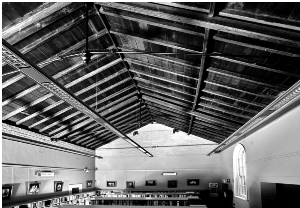
The remaining section of the School of Arts hall after the conversion in 2007 - showing the original timber-planked roof lining, the iron bracing, and on the right, one of the original windows
