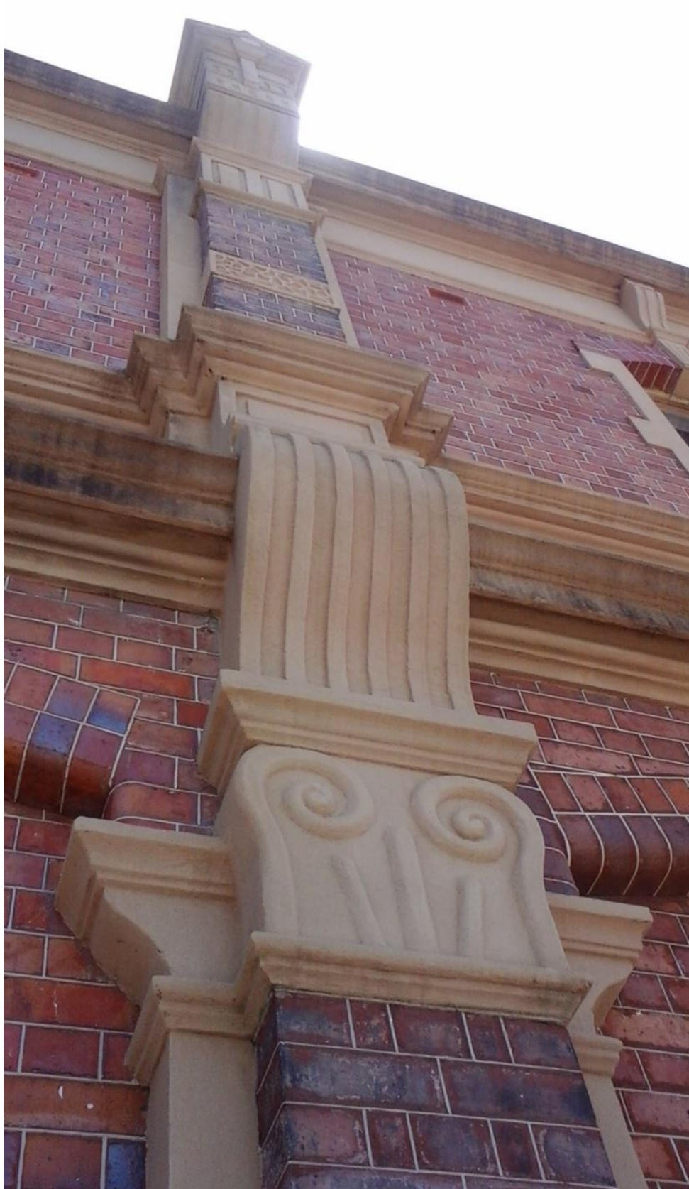
Detailed close-up of pilaster higher on the building depicting the idiochromatic nature of the brickwork and the ornately varied cement work. Photo Sally Henning.
