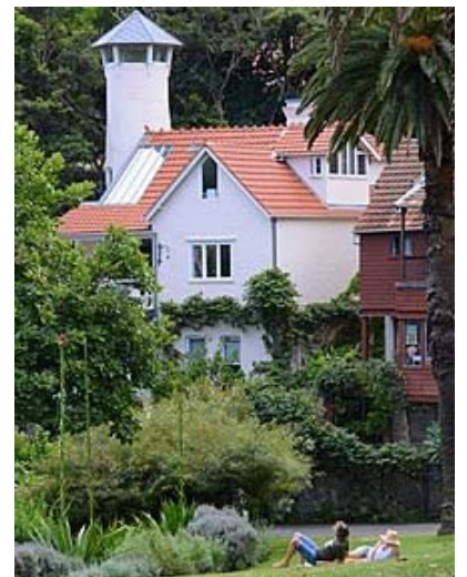
The Whiteley home at lavender Bay
